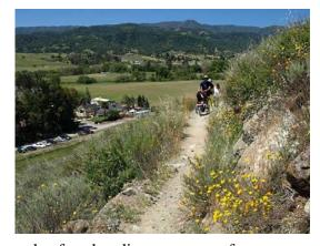
Note that a trail bed of 4 feet does not mean that the trail tread, that portion of the trail that is normally walked or ridden on, need be a full 4 feet. Most trails will fill in with vegetation leaving a 1 to 2 foot tread but will still have room for passing.
